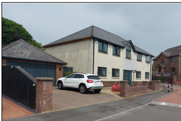
Figure 2 Photograph of existing front elevation
